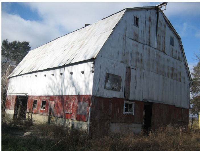
The gambrel roof with vertical walls appeared in the second half of the nineteenth century as a solution to the need for greater storage space.
