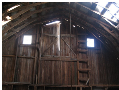
The gambrel roof with vertical walls appeared in the second half of the nineteenth century as a solution to the need for greater storage space.
