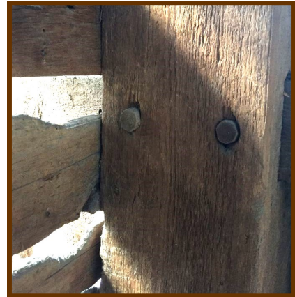
Pegs holding the timbers together
