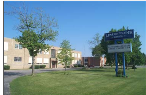
Limestone Elementary School serves “county west”
