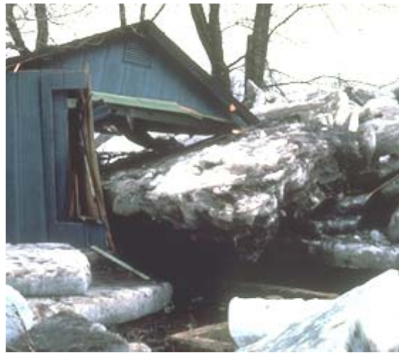
Kankakee River ice jam damage, 1982
