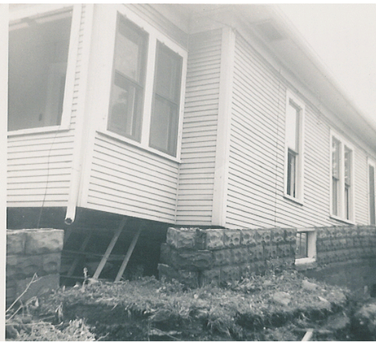
Soldier Creek flood damage, 1957
