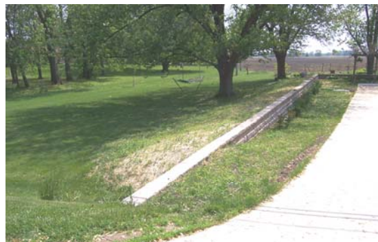
This barrier in Otto Township protects the home from flooding from the stream to the left.
