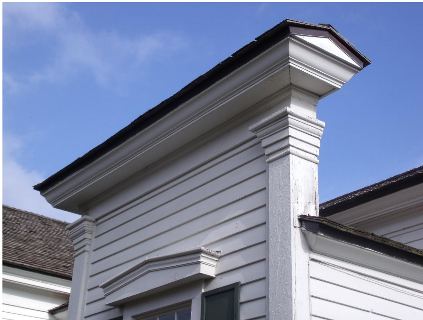
This heavy cornice can be seen on the east southeast corner of the house. A cornice is the uppermost section of moldings along the top of a wall or just below a roof.
